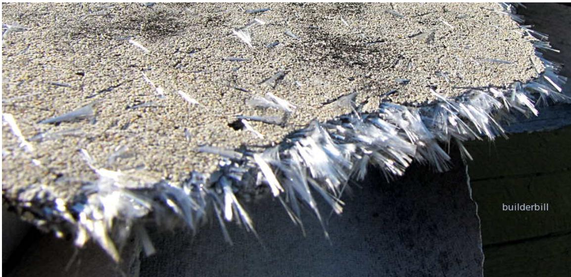
Img 5.13: Part of a “Super Six” roof hip flashing that is severely weathered. ACM like this in my opinion falls into the classification of Friable asbestos. The asbestos fibres are no longer firmly bonded into the cement mix. Note that the surface cement paste has eroded away showing the individual grains of sand.
