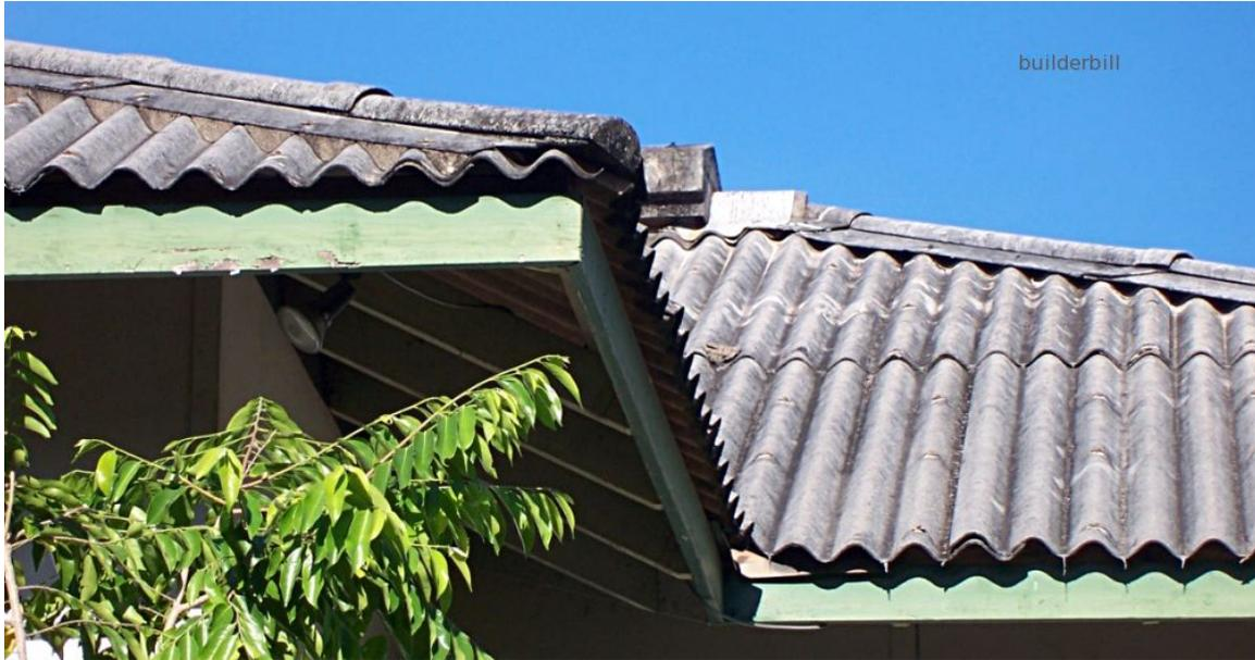
Img 5.11: “Super Six” corrugated sheeting. Produced by James Hardy & Co. In Australia. This photograph shows a roof dating back to the 1950’s. The left hip flashing uses cement mortar to seal the gaps, which is not unusual, particularly on lower pitched roofs. It is just possible to see the end of an AC ridge vent which were used a lot on these roofs.
