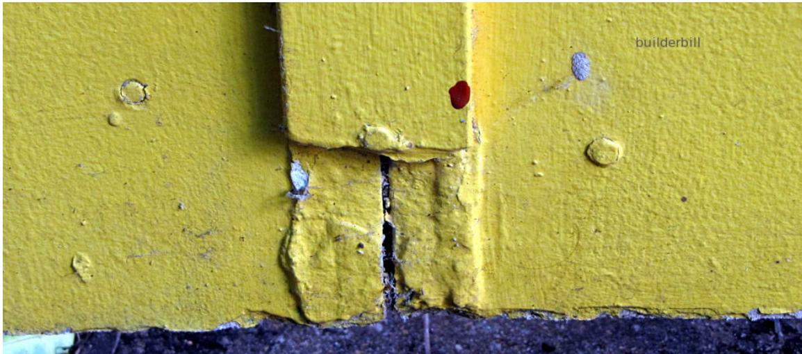
Img 5.2: Flat sheet cover batten with typical broken end.
