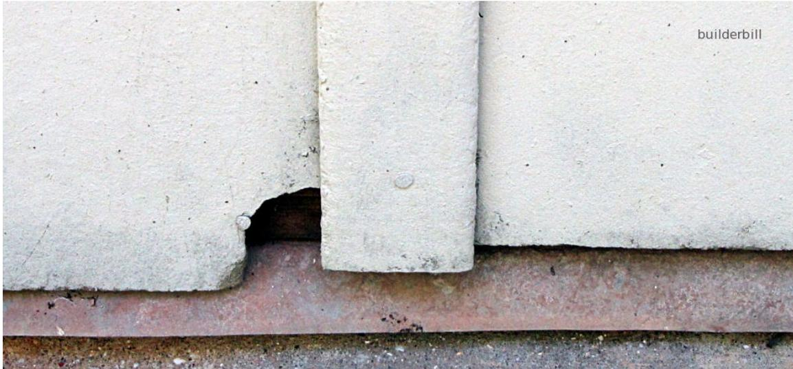
Img 5.6: Another typical corner break in an AC sheet
