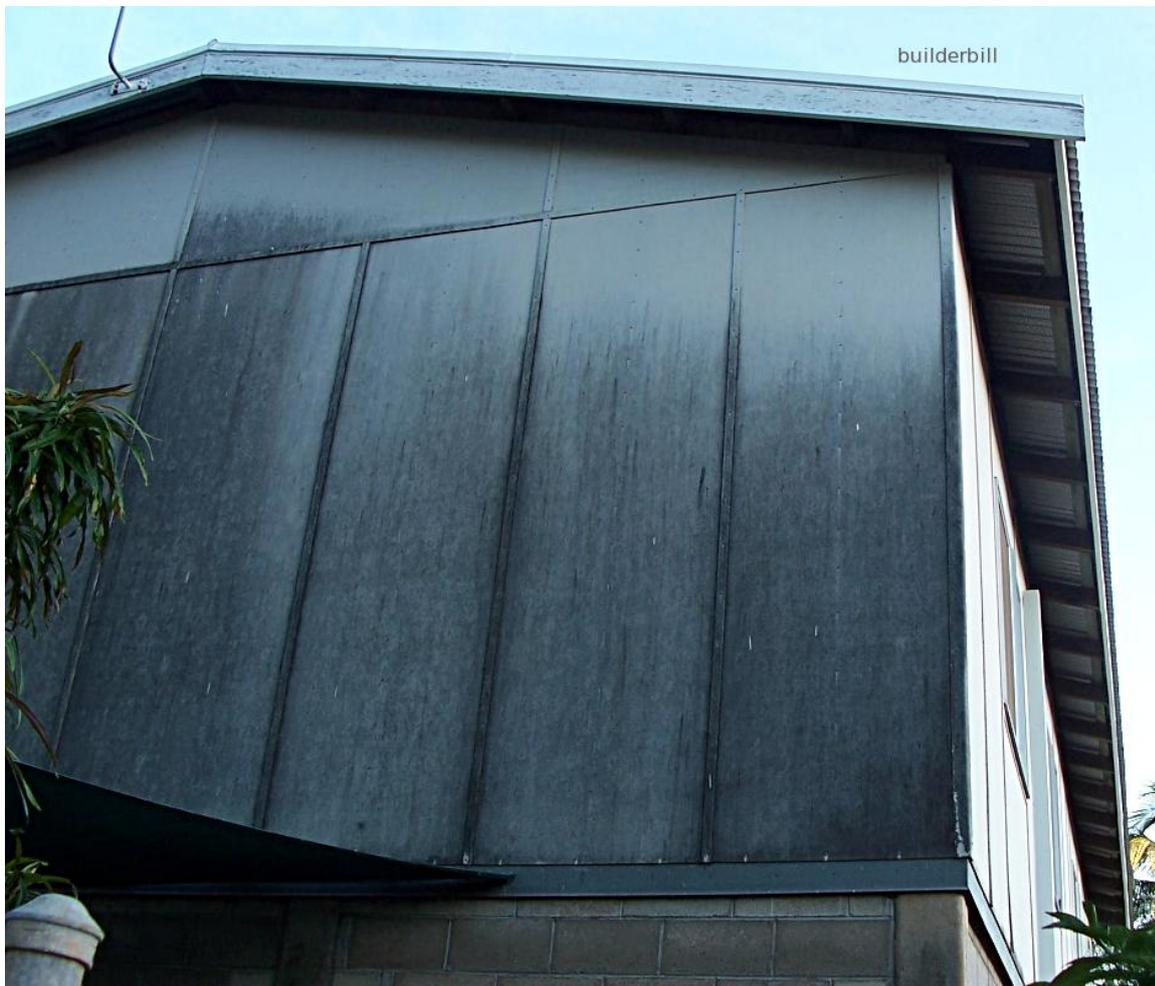
Img 5.1: An elevated timber frame house clad with AC flat sheets. The horizontal batten at the gable triangle hides a small “Z” type flashing that sits under the top sheets and under the bottom ones. The dark mildew type staining is typical of unpainted AC sheets.
