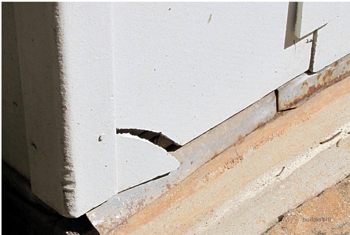
Img 5.5: Typical break in sheet where the nail was too close to the edge of the sheet. (The nail did not break the corner mould because these were generally thicker and had more asbestos fibre reinforcing than the flat sheets)
